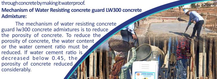
If we further reduce the water/cement ratio, the workability of concrete decreases. This can be prevented by the use of concrete guard lw300 waterproofing concrete admixture that ensure sufficient workability of concrete for full compaction and reduce shrinkage cracking.
